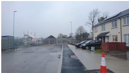
Figure 18.11: View of housing under construction, north boundary of proposed southern site.
